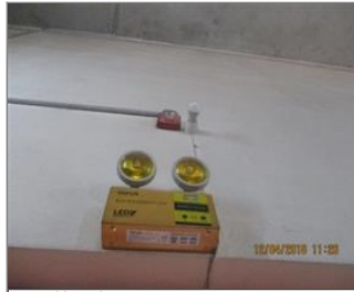
Photo of fire safety equipment Fire bell.JPG
