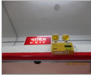
Photo of fire safety equipment Exit sign illuminated.JPG
